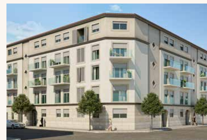
Edificio Major, Lluç major, Mallorca
